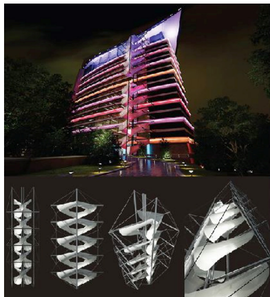
Emergency Evacuation Systems in High-Rise Buildings. Image: UNAM - Structures Laboratory archive
