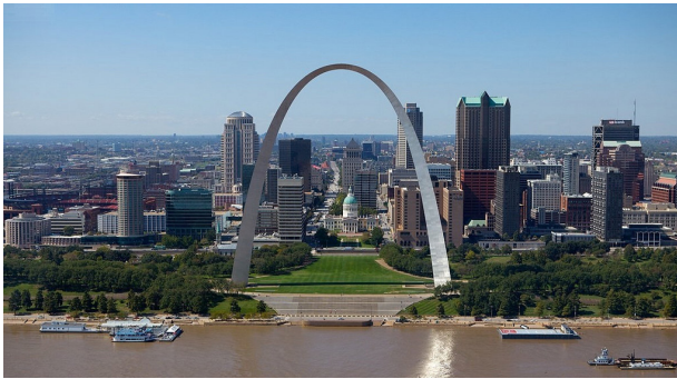
Example of the relationship between form and structural behavior. Image: Sam Valadi, Gateway Arch , flickr.com.
