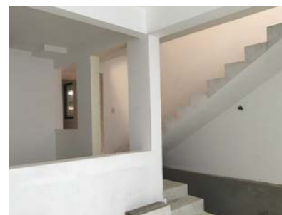
Figure 4: Walls and ceilings covered with gypsum plaster.
