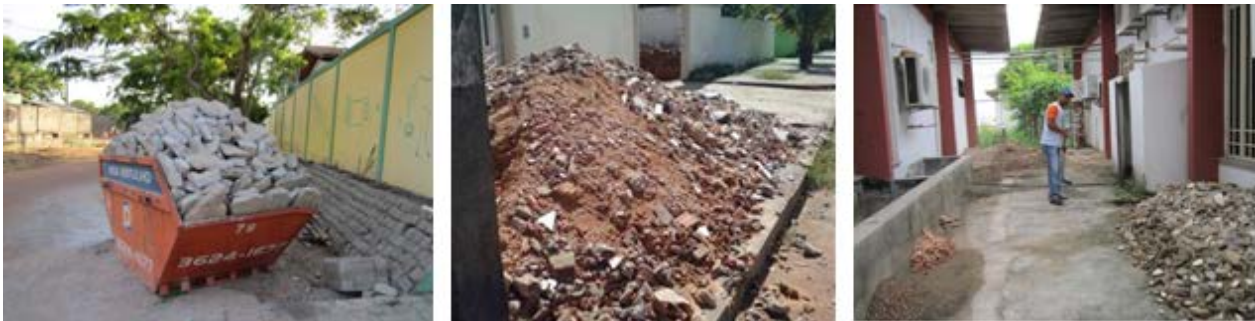
Figure 5. Collection and disposal of CDW.
