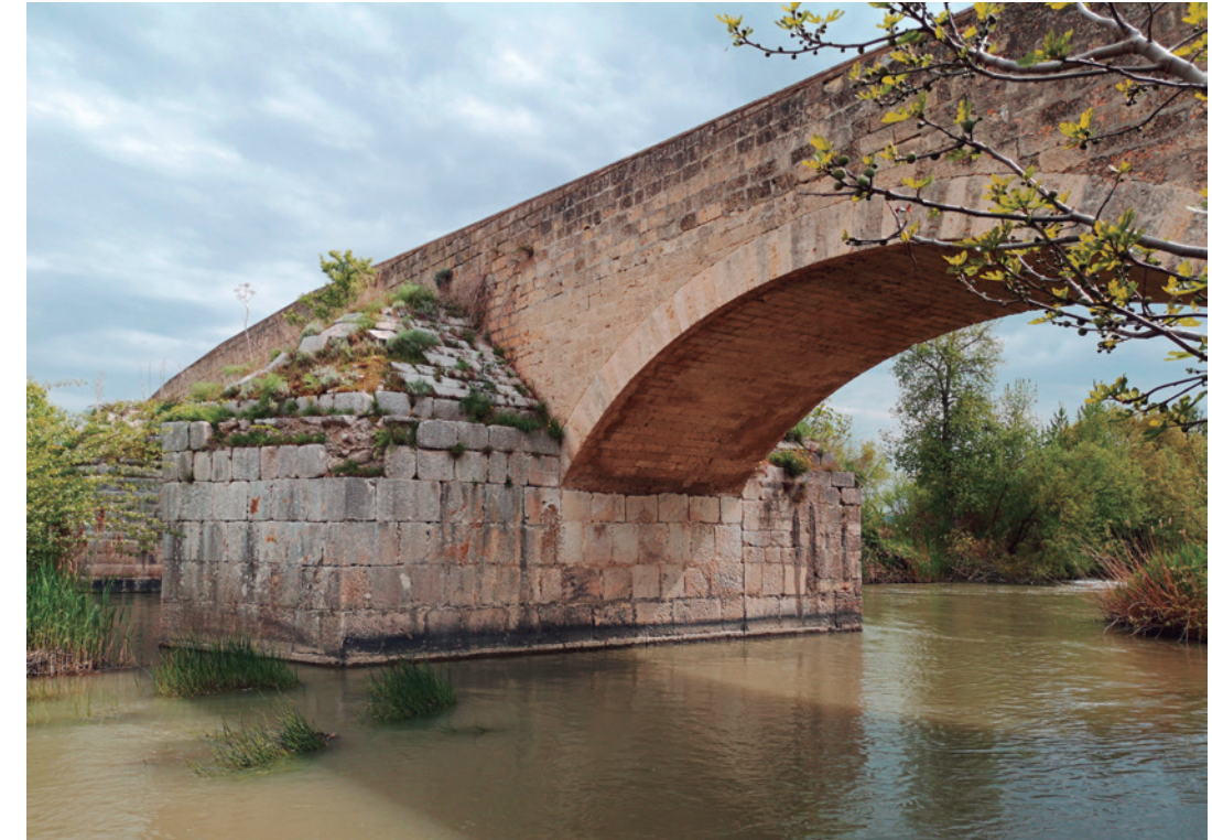
View of the bridge from the west bank (detail), Canosa di Puglia, 2019. Photograph: Germano Germanò
